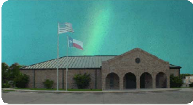
Southmost Community Network Center
